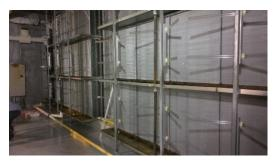
These are used for controlling microbial growth on cooling coils<sup>i</sup> and is also helpful with disinfecting air as it is supplied to rooms and areas inside buildings.
